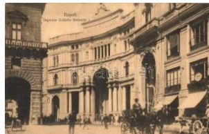
21833. ☒ Naples, Napoli; In gresso Galleria Umbert 1600
