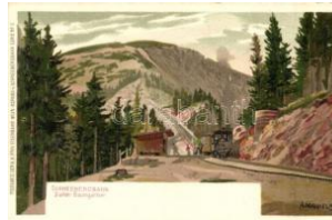
21589. Schneebergbahn, Station Baumgartner 2400
