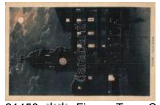
21450. ** Fiume, Torre Civica / civic tower at nig 1000
