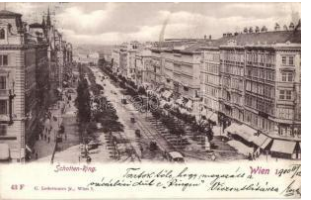
21382. ☒ Vienna, Wien I. Schottenring / street, tram 1000
