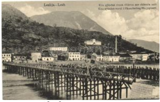
21254. ** Lezhja-Lesh, te mporary bridge with so 2000
