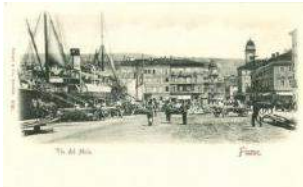
21160. ** Fiume, Via del M olo / ship station T1 1600
