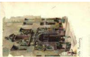
21640. ** München, Alte Residenz / old residence 1800
