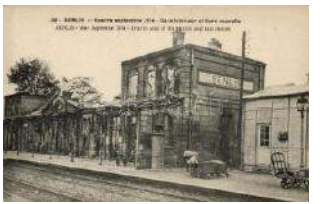
21536. 1914 Senlis, Interior side of the station an 4400
