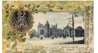
21595. ☒ Altona, Hauptbahnhof / railway station, c 3000
