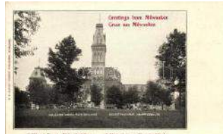
21277. ** Milwaukee, Wisconsin; Soldier's Home, Main Build 2000
