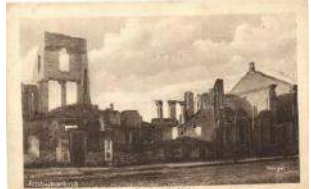
21385. ☒ Brest-Litovsk, War damaged buildings T2 2600
