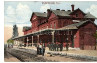
21536. Marasesti, Gara / railway station (EK) T2 3000
