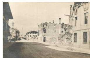
21466. * 1918 Palmanova, WWI destroyed building 1800
