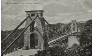
21366. ** Bristol, Clifton Suspension Bridge; Delittle 800
