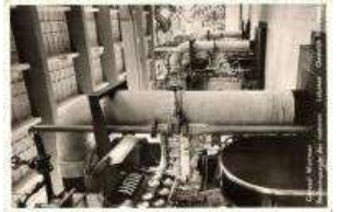
22474. ☒ Lelystad, Gemaa l Wortman / pumping st 1000
