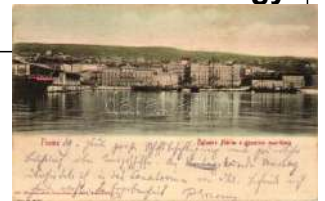
22001. ☒ Fiume, Adria palota / Adria Palace, marit 1400
