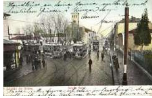
22728. * Braila, Strada Galati / street view with tram 2600
