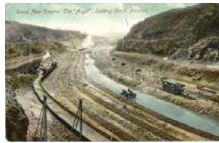
21836. * Panama, Canal near Empire, The Angle 1800
