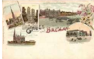
21609. ** Wrocław, Breslau; Lessingbrücke, Schw 4000
