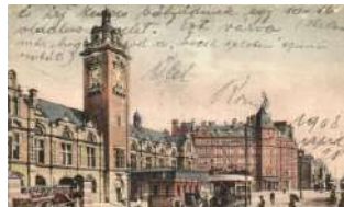
21637. Nottingham, Victoria Station, tram (EK) T 2000
