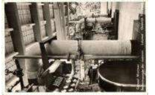
21865. ☒ Lelystad, Gemaa l Wortman / pumping st 1000
