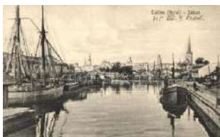
21802. ☒ Tallinn, Reval; Sa dam / port, steamship ( 1000
