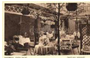
21899. ** Katowice, Katowice; Hotel Savoy, Ogród 2400
