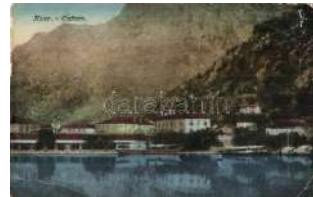
22253. ☒ Kotor, Cattaro; P ort, general view (EB) T3 800
