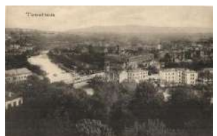
22243. ** Cieszyn, Teschen; general view, river, 2200
