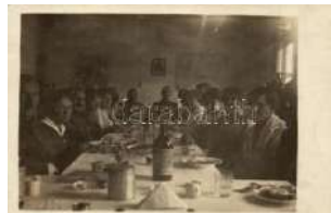
21362. ☒ Cetinje, Hospital dining room, photo. K.u 3000
