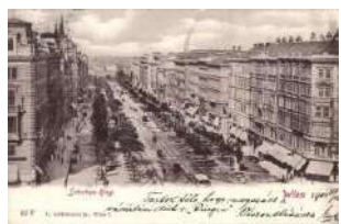
21334. Vienna, Wien I. Schottenring / street, tram 1000
