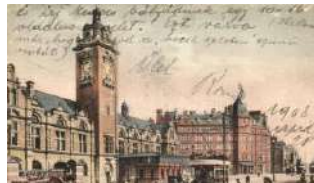
21561. ☒ Nottingham, Victoria Station, tram (EK) T 2000
