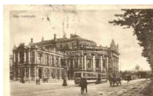
21895. ☒ Vienna, Wien; Burgtheater / theatre, tram 1200
