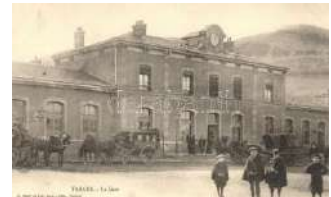
21998. ** Tarare, La Gare / railway station T1/2 3000
