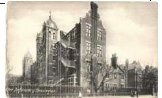
22074. ** Kensington, The Infirmary, hospital (from 2000)
