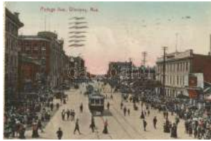
22016. ☐ Winnipeg, Portage Avenue, tram, shops 1000
