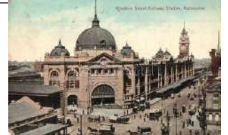
21818. ☒ Melbourne, Flinders street railway station 2000
