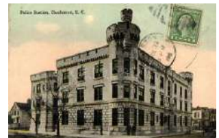
21606. Charleston, Police Station (EB) T3 2200
