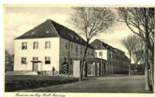
21800. ☒ Freising, Kaserne-des Erg. Batl. / barrack 1800
