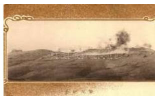
22153. ** Blowing up of S unghushan fort, Japan 3000
