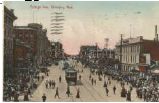
21748. ☒ Winnipeg, Portage Avenue, tram, shops 1000
