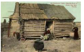
21611. Florida, Old Fash ioned Cabin Chimney B 2400
