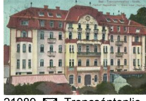
21089. Trencsénteplic, Trencianske Teplice; Tep1200
