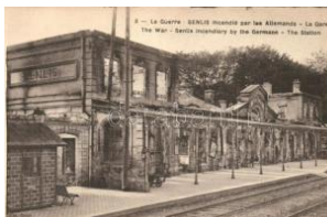
21312. Senlis, Railway station destroyed by th 4000
