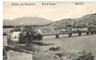
22109. ✱✱ Shkodër, Shkodra; bridge T1 2400
