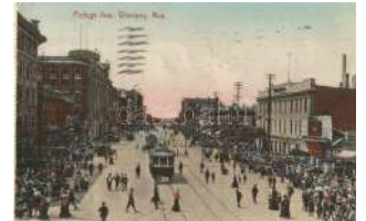
22321. Winnipeg, Portag e Avenue, tram, shops 1000
