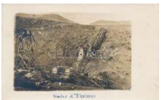
22306. 1917 Eksi Su, Eks issou; Blown up bridge 3000
