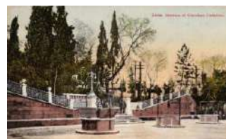
21973. ✱✱ Zadar, Zara; entry of the Public Garden 1400
