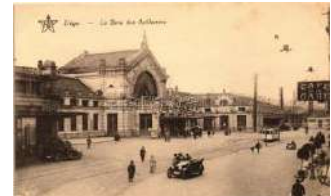
22209. ** Liege-Guillemin s railway station, cafe, 2000
