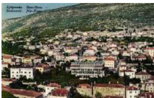
21925. ** Dubrovnik, Pile Kono T1/2 1200
