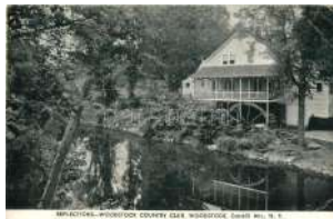
21751. ✱ Woodstock, County Club, water mill (EK 1000
