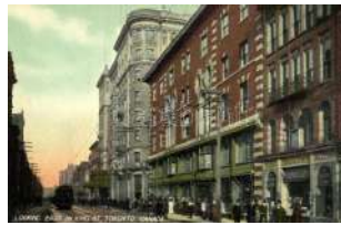
21865. ** Toronto, Looking east on King Street, Toronto 2000
