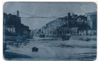
22101. Bristol, Clifton S uspension Bridge T2 1400
