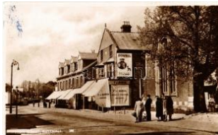
22350. ☒ 1957 Rusthall, High Street, shop of F.J. 2000
