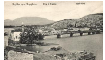
22212. Shkodër, Shkodra; bridge T1 2400
