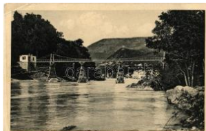
22635. ✱ Solkan, Salcano , Most cez Soco / bridge 2000
