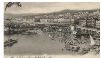
22228. Algiers, Alger; port, Boulevards (EK) T2/ 1000
