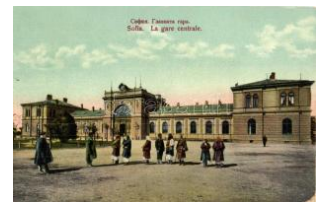
22296. * Sofia, Sofia; La gare centrale / railway station 2000
