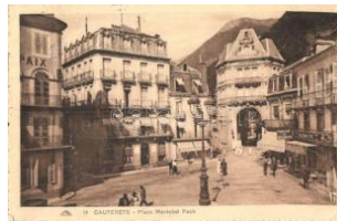
22319. ☒ Cauterets, Place Marechal Foch, Salon d 1400
