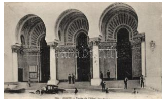
22222. Algiers, Alger; Entrance of the Hotel des Postes 1400
