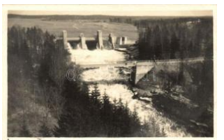
22159. ** Imatra, river dam, bridge T2 1400
