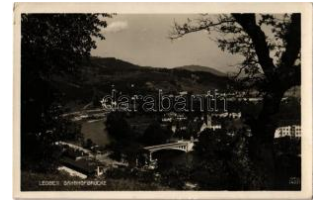
22022. ☒ Leoben, Bahnhofbrücke / railway station 1400
