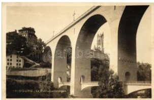
22331. ** Fribourg, Zaehringen bridge T1/2 1200
