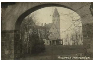
22138. * 1927 Taagepera, Sanatorium, photo T 2000
