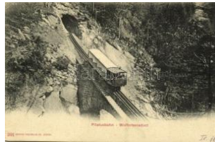
22576. ✳✳ Pilatusbahn, Wolfertsviaduct / cog T2/31000
