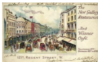
22272. * 1911 The New Gallery Restaurant a T2/32000
