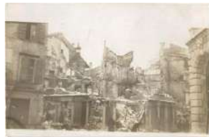
23811. ** Udine, WWI de struction, house ru T1/2 2600
