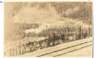
23525. ** Lower Spiral Tunnel, Field, Canada T1/2 2000
