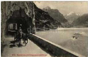
23910. ** Bristenstock, Axenstrasse / road T2 T2 1000
