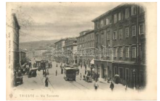
23122. Trieste, Via Torre / street view, tr T2/3 2600
