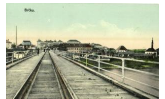
22854. ☒ 1909 Brcko, Brck; railway bridge / Ei T2 3000
