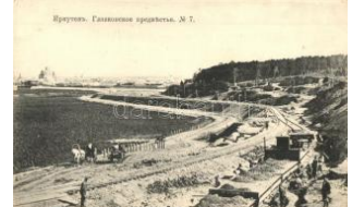
23130. ** Irkutsk, construction of railways, rail T2 2400
