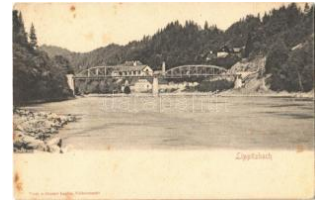
22810. ** Lippitzbach, Brücke / bridge (fl) T2/ T2/3 1000
