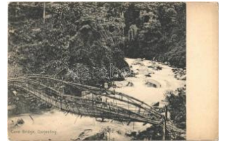
22942. Darjeeling, Can e Bridge (fi) T2/3 T2/3 1000
