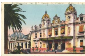
22979. Monte-Carlo, Le Casino / The Casin T2/31600
