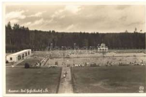
22437. Grofsröhrdorf, Massenei-Bad / spa, T1/2 2000
