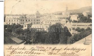
22148. * Bad Vöslau (wet damage) T3 T3 1400
