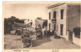
22350. * Medenine, La Poste / post office, aut T1/2 2000
