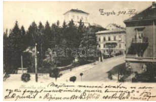
21769. Zagreb, Mesnicka ulica / street view T2 T22400
