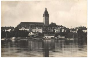
22308. ** Strangnas, general view, church, T1/2 2000
