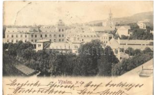
21861. * Bad Vöslau (wet damage) T3 T3 1400
