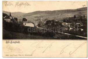
22342. 1902 Altlenzbach, general view T2 T2 1000
