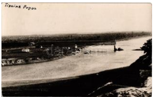
22120. * Tighina, Bender; Podul / destroyed railw T 5000
