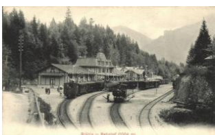
22155. * Brünig, Bahnhof / railway station wit T2/3 2800
