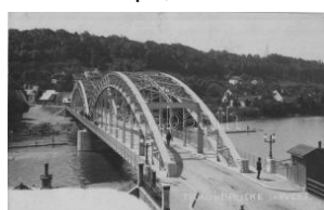
21653. ✱✱ 1901 Wels, Traunbrücke / bridge, tim T2800
