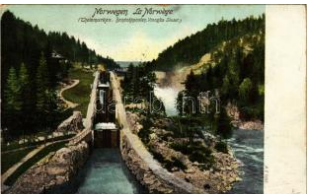
22314. 1904 Telemarken, Bandakkanalen, V T2/31000
