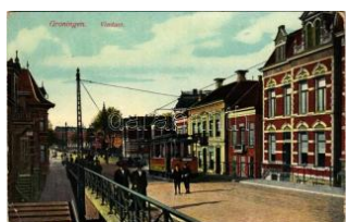
22095. ** Groningen, Viaduct / bridge, tram ( T2/3 1600
