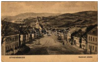
21918. 1914 Strengberg, street view, church. Jos T2/3 1800
