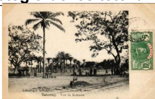
22394. ✱ Bohicon, Vue / general view, railway T1 3000
