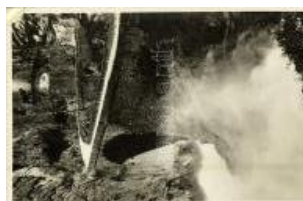
23302. 1937 Andermatt, Teufelsbrücke / bridge T3/800
