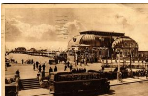
22790. 1936 Worthing (West Sussex), Pier & P T3 1000
