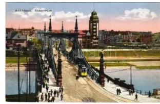
22299. Mannheim, Nec karbrücke / bridge, tr T21600
