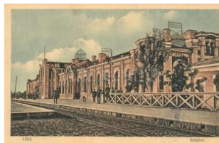
22145. Lida, Bahnhof / railway station (EK) T T2/3 4000
