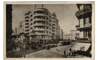
22199. ☒ 1949 Cairo, stree t view, tram, autom T2/31000
