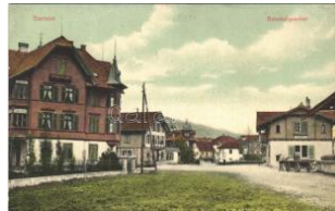
21960. ** Sarnen, Bahnhofquartier / railway s T1/21400
