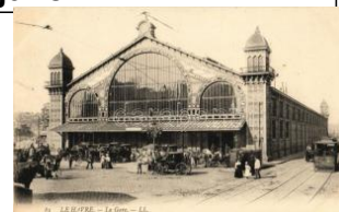
22381. ** Le Havre, La Gare / railway station, T21000
