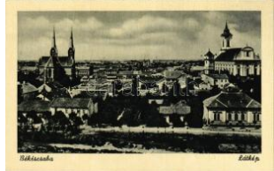
20195. *** Békéscsaba (áz ott / wet damage) T T2/31000
