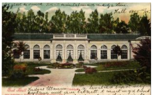
22526. ☒ 1905 Bad Hall, T rinkhalle / drinking ha T21600
