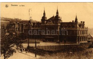
22666. 1933 Verviers, La Gare / railway stat T2/3 1000
