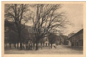
21896. ✱✱ Trencséntepic, Trencianske Teplice T21800
