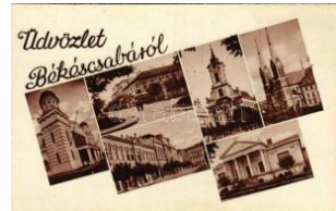
20193. *** Békéscsaba (áz ott / wet damage) T T2/31000
