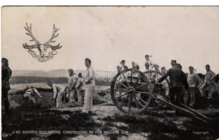
24014. ✱✱ 2nd Seaforth Highlanders construct T3 1000
