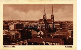
20194. *** Békéscsaba (áz ott / wet damage) T T2/31000
