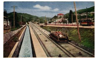
22877. * 1929 Kyoto, The Osui (canal) incline T2/32000
