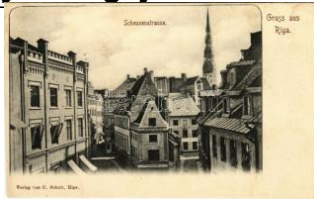
22907. * Riga, Scheunenst rasse / street view. T2/3 1600
