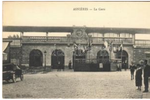
22910. ** Asnières-sur-Seine, La Gare / railwa T2 1600
