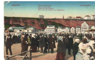
22942. 1916 Helgoland, Landungsbrücke / T2/3 1400
