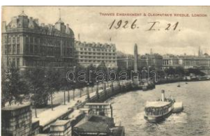
22927. ☒ 1926 London, Thames Embankment T2/3 1000
