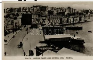
22901. ** Sliema, Landing place and general T1/2 1000
