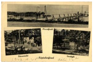
20911. ☒ Káptalanfüred (B. alatonalmádi), Stra T2/31600
