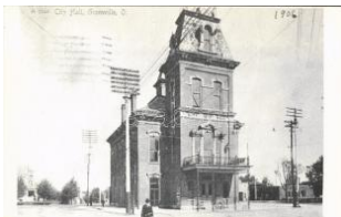
22615. ** Greenville (Ohio), city hall T1 T1 1000
