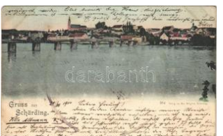
23184. 1900 Schärding, general view, bridge T3/41000
