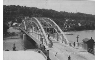
23195. 1901 Wels, Traunbrücke / bridge, tim T2/600
