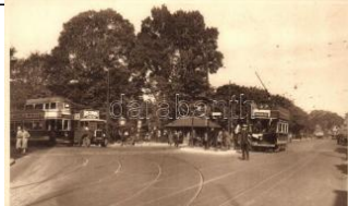
22434. ** Southampton, Junction Corner, tram T1 3000
