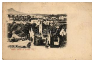
22079. 1903 Port Arthur (Tasmania) genera T2/31000
