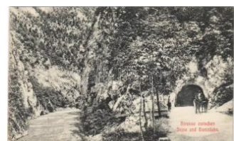
22164. Banja Luka, Banjaluka; Strasse zwis T21000
