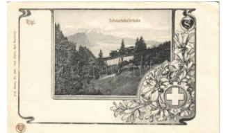
22780. ** Rigi, Rigibahn; Schnurtobelbrücke T2/31000
