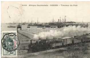
22785. ✳ Dakar, Travaux de Port / Port works w T25000
