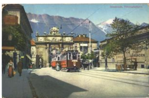
21958. ☒ Innsbruck, Trium phpforte / tram, str T2/3 1600
