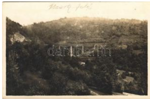
22584. * Uzsok, Uzhok; St erbinsky viadukt / v T2/32800
