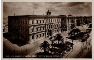
23035. ** Bari, Via Cavour, Palazzo delle Post T1/2800
