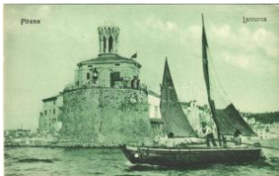
23163. ** Piran, Pirano; L'antenna / lighthouse, T2 2800
