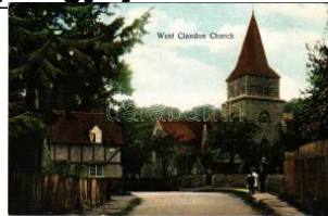
22586. ** West Clandon, Church, street view T2/3)1000
