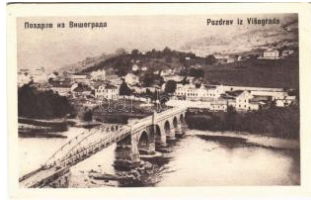
22437. ** Visegrad, general view, bridge (EK) T2/3 1000
