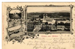
22614. ☒ 1905 Metten, general view, church, ca T3)2000
