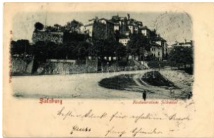
22439. ☒ 1899 Salzburg, Restauration Schanzl T2 1600
