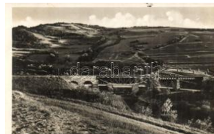
22165. Uzhok, v iadukt / viaduct T2 T2 1400
