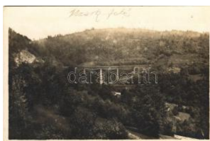
22718. * Uzsok, Uzhok; St erbinsky viadukt / v T2/32800
