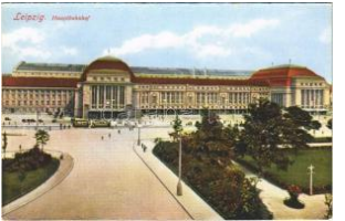
23016. ** Leipzig, Hauptbahnhof / railway station T11000
