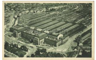
23015. ** Leipzig, Hauptbahnhof / railway station T1/21600
