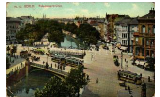
22983. 1908 Berlin, Potsdamerbrücke / bridge, T31600
