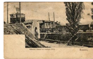
20639. ✱ Budapest XXII. Bu dafok, Villamos viadu T43200
