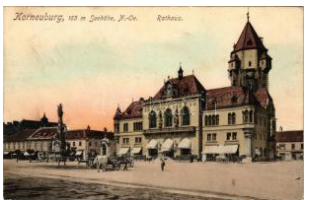
22803. 1917 Korneuburg, Rathaus / town hall T2/3 2000
