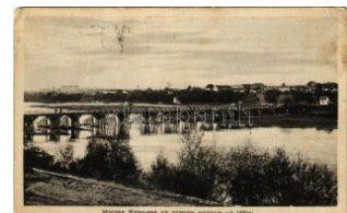
23126. ✱ Kraljevo, old bridge on the Ibar (EK) T2/3 1000
