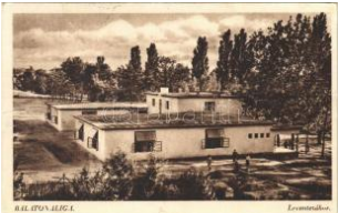
20180. ☒ Balatonakali, Balatonvilágos, Leve T3/4 1200
