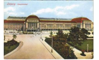
23339. ** Leipzig, Hauptbahnhof / railway station T 800
