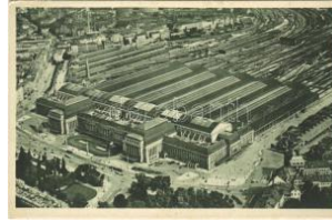
23338. ** Leipzig, Hauptbahnhof / railway station T1/2800
