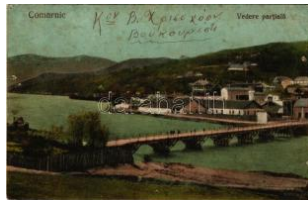
24158. * Comarnic, Komarnik; bridge (pinhole T3/42000)
