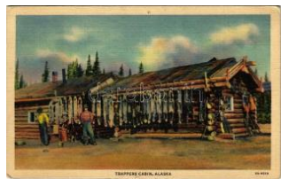
23328. 1940 Alaska, Tra ppers Cabin (pinhole) T41000
