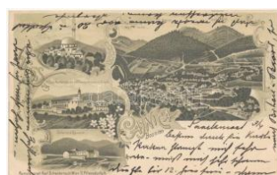
23388. ☐ 1902 Cajnice, Caenica; Montenegro T210000
