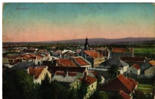
23344. ** Amstetten, general view T3 T3 1000
