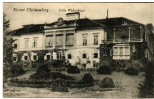
22848. Bad Gleichenberg, Villa Wickenburg T1/2 1600
