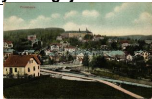
22903. Pressbaum, general view, bridge (EK T2/31600)
