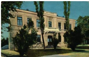
23198. * Braila, Administration Building Bailor Lacului S T2/3 1000
