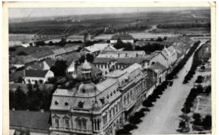
22895. * Zenta, Senta; Vas hid / iron bridge T31200
