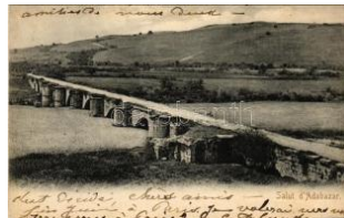
22959. * Adapazari, Adabazar; Roman bridge (b) T41000
