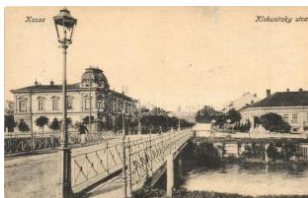
21640. * Kassa, Kosice; Kl obusitzky utca, híd T1/2 2200
